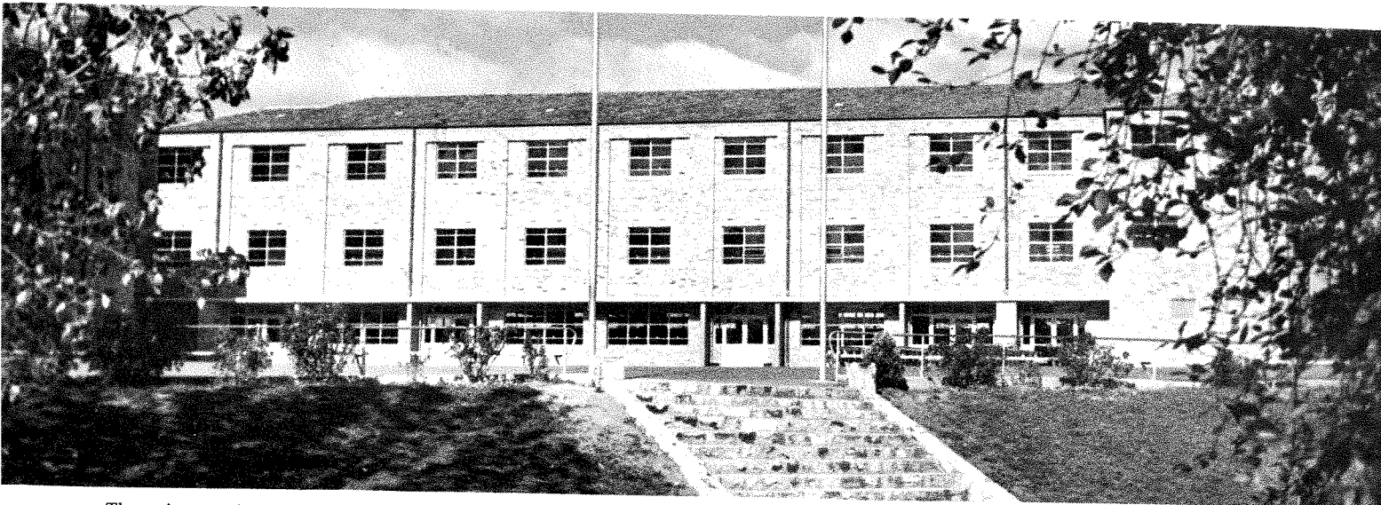
The science wing, completed in 1966, contains Physics, Chemistry and Biology laboratories, two demonstration rooms, three General Science rooms, six preparation rooms, one workshop and one plant room. The basement contains the tuckshop and bookroom and a large assembly area.
